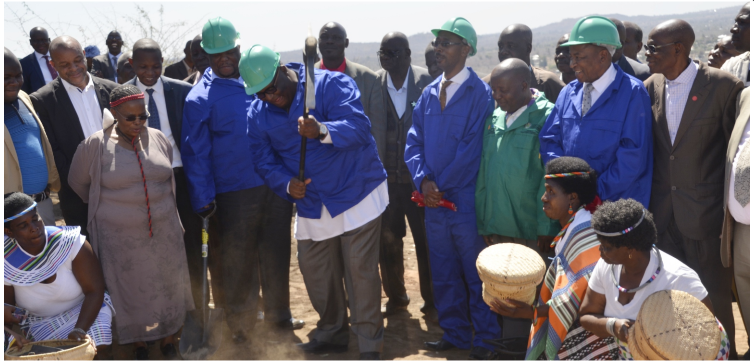
MEC Ndou officially declares the commencement of the construction of Masia Traditional Council offices.
